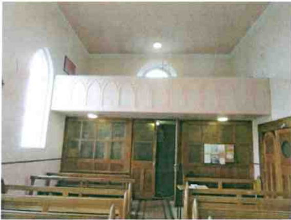
Repositioning of inner entrance screen should be considered
