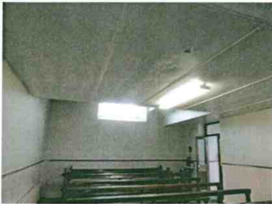
Soffits to Galleries to be replaced
